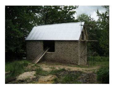
spell of dry weather in which to carry out the main work – re-roofing the barn and repointing the walls. The work was carried out by specialists in the repair of old buildings, the Bucknall Partnership from Colyton."
